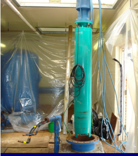
250 HP Indar being installed in Brookfield, WI
